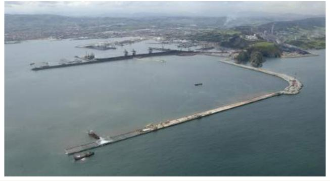
Figure 123: Construction works of rubble mound and vertical breakwaters in Gijon Port (Spain)
