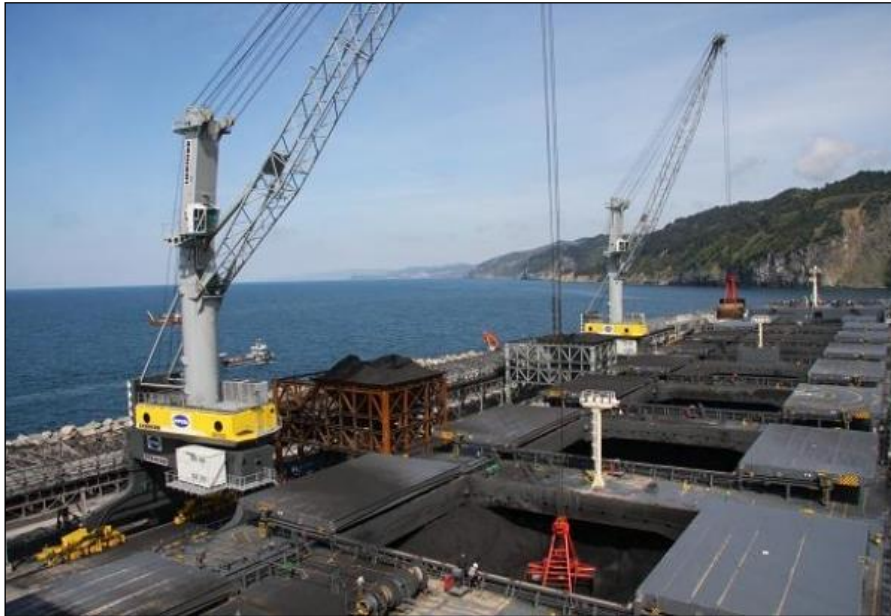
Figure 7.8 Typical Mobile Harbour Cranes with Mobile Hoppers
