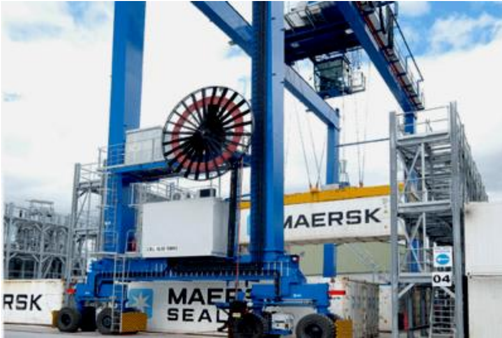
Figure 7.10 Typical E-RTG for Yard Operation
