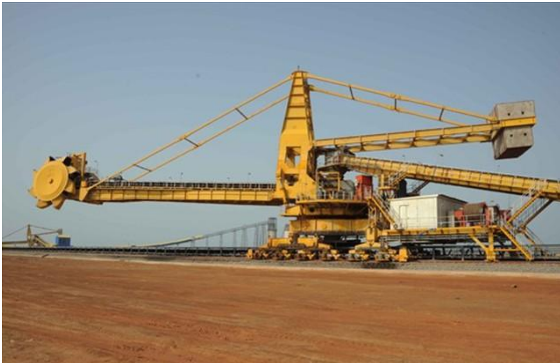
Figure 7.2 Typical Stacker cum Reclaimer
