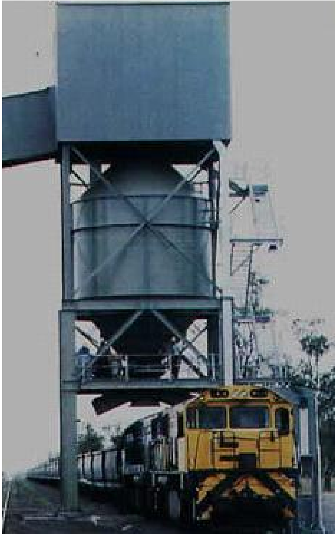
Figure 7.3 Typical in-motion Wagon Loading System
