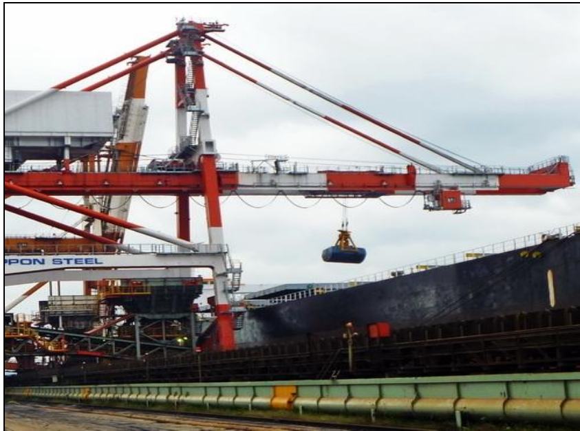
Figure 7.1 Typical Gantry Type Ship Unloader
