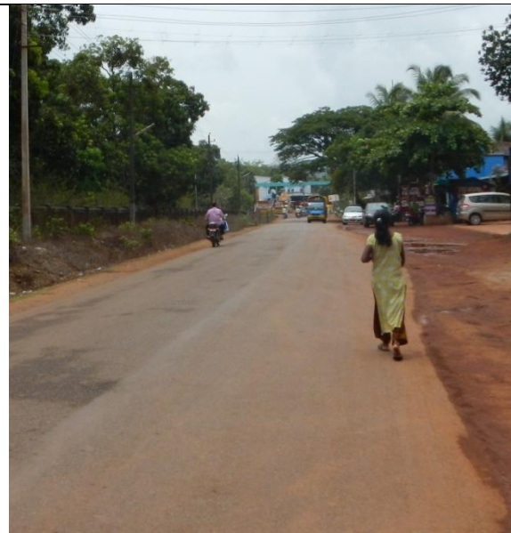
Dr. Dinaker Desai Road (7 m) connecting Ankola to NH 17; 1 km stretch; commercial establishments and habitation on both sides
