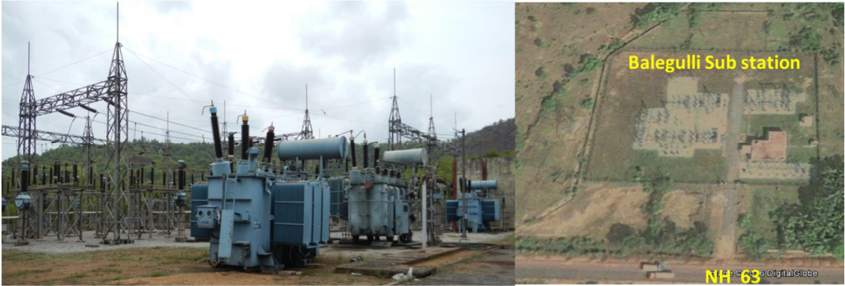
Figure 2.16 Location of Balegulli Substation
