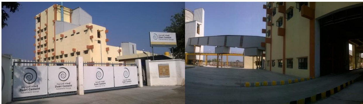
Figure 8.4 Zuari Automated Cement Plant at Ernakulam Wharf (Q5)
