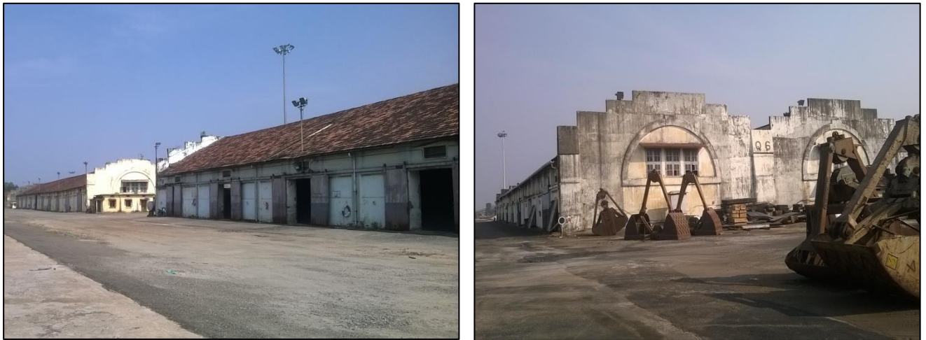
Figure 3.5 Storage Sheds at Mattanchery and Ernakulam Wharf
