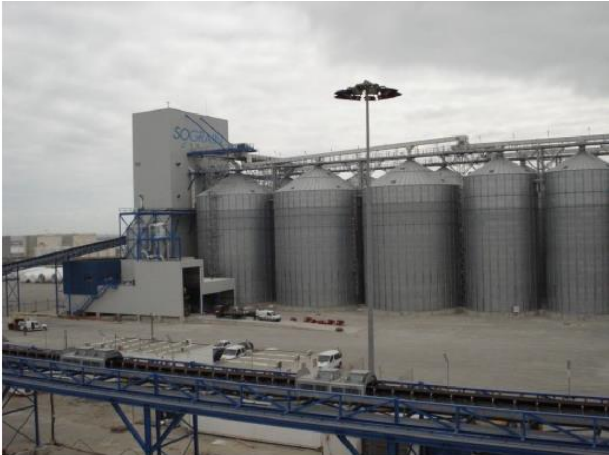
Figure 8.2 Steel Silos for Food Grains
