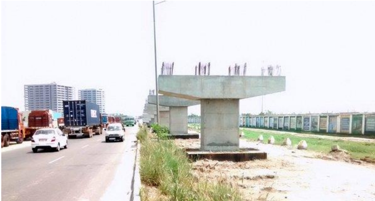
Figure 5.4 Construction of ROB to Ease Congestion
